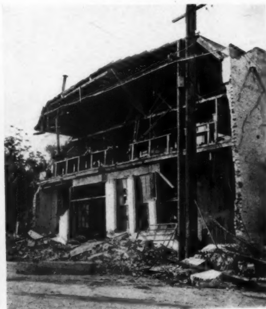
FIG. 6. TYPICAL DESTRUCTION OF BRICK FRONT
